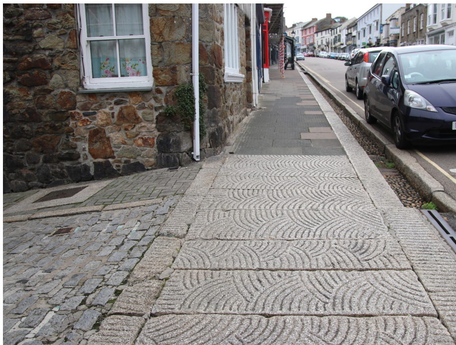
Coinagehall Street. The entrance to Lady Street is on the left and the kennel running down this street can be seen to the right of the pavement. The granite paving here is grooved to provide both decoration and resistance to slipping.
