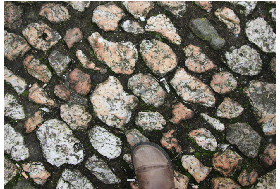
Veinstone, the waste product of metal mining which makes hard-wearing cobblestones that are used for paving in various localities in the town of Helston. It is best seen at Five Wells and outside the Band Room on Church Street.
